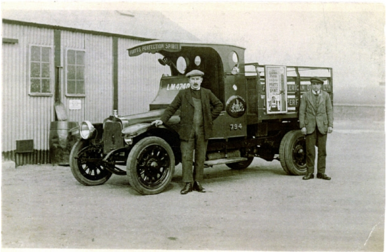
Pratts had a filling plant at their Sandwich depot (above) where all empty cans had their tops repainted and new leather washers inserted into the brass screw caps before being refilled. The smaller depots, including Ramsgate, were closed around 1936. In this picture is Alf Miller with his driver's mate Sid Finch.
